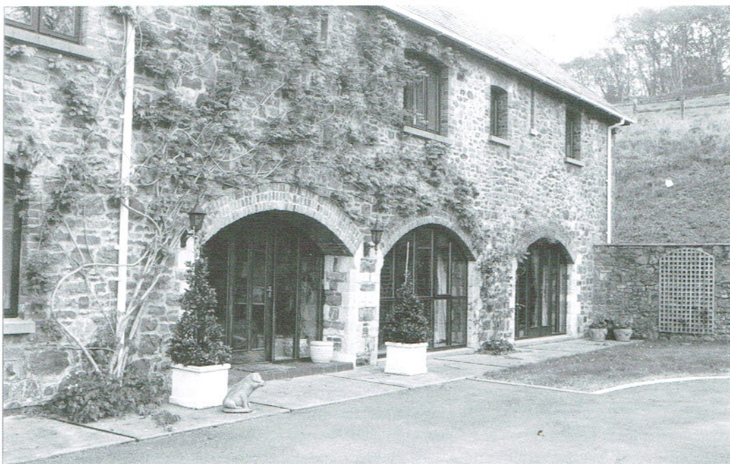
Fig. 30. The south wall of the Home Farm (the re-used medieval oolite quoins can be clearly seen).
