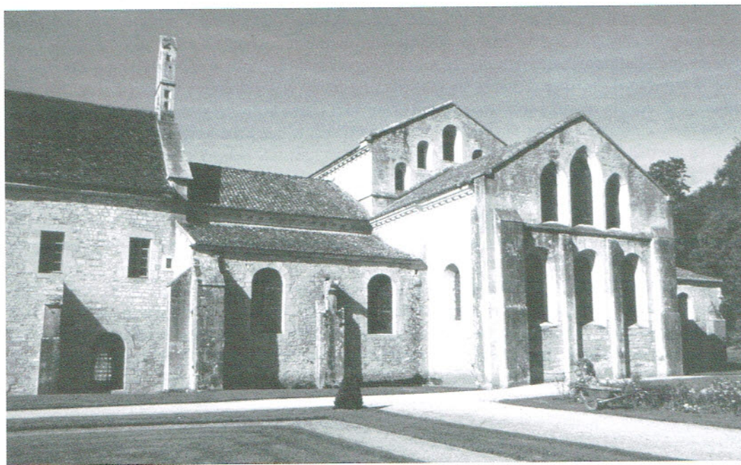
Fig. 8. The east end at Fontenay Abbey (Burgundy), before recent alteration of the lean-to chapel roofs into gables. Photograph: David Robinson, English Heritage.
